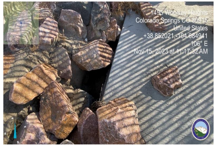
Photo 6: North riprap at gutter pan has visible voids, fill voids to eliminate chance of erosion.
