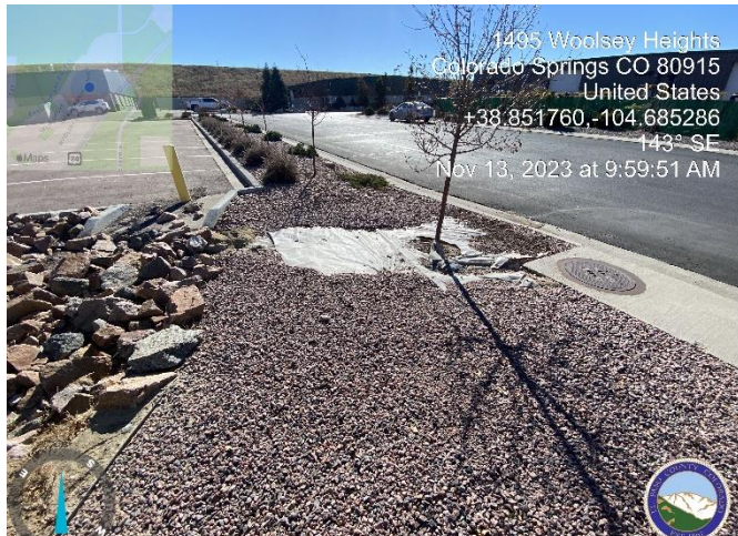
Photo 1: Erosion control mat not installed at southern perimeter of pond at spillway. In an overflow event the landscape rock will (and already has) washed out
