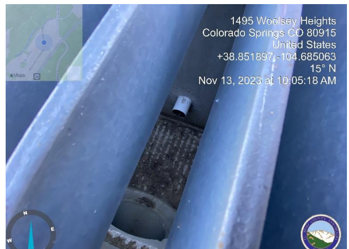
Photo 4: Orifice at underdrain outlet not installed.
