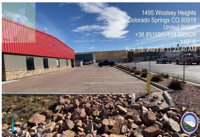
Photo 7: 6' concrete gutter pan not installed in southern parking lot.
