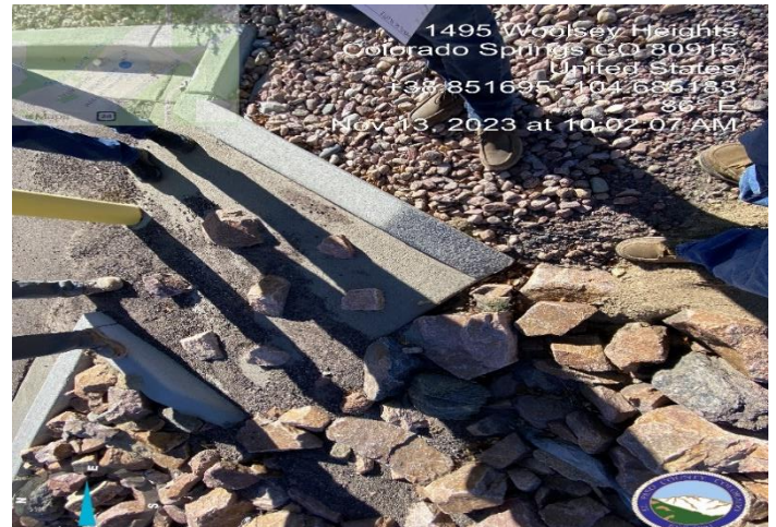
Photo 2: Rock present in gutter pan, reflect this on as-builts
