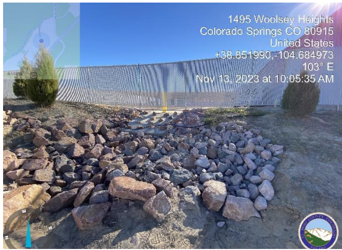
Photo 5: North riprap type VL not installed at 24.5 feet (9 feet short). Install per plan or if M&S is ok with it as-is, reflect this change on the as-builts
