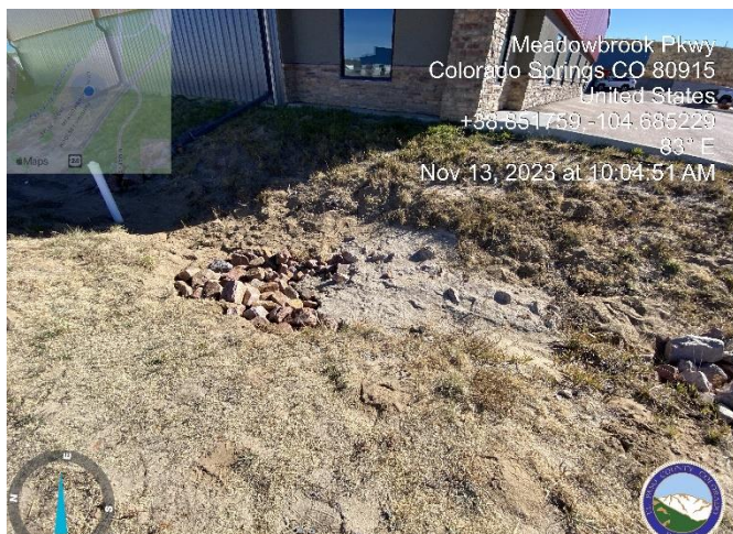
Photo 3: Excess rip rap and concrete near southern 4" underdrain. Evidence of previous undercutting north of the southern riprap rundown. Extend riprap to pond bottom
