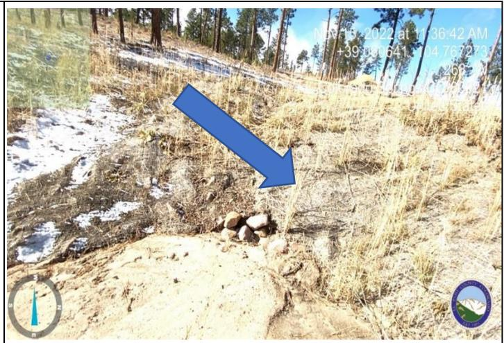
Photo 2: Confirm that soil riprap was installed per spec for Pond A1 is installed
