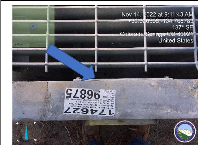
Photo 1: Pond A1, Pond C1, and Pond C2) are missing gaskets between orifice plate and outlet structure
