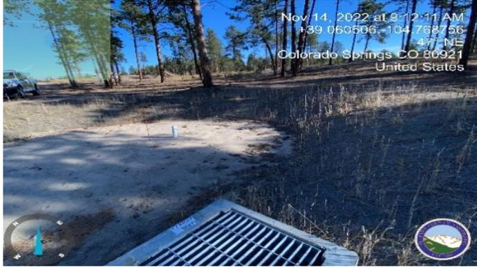
Photo 5: Sparse vegetation on embankments of Pond A1, Pond C1, and Pond C2.
