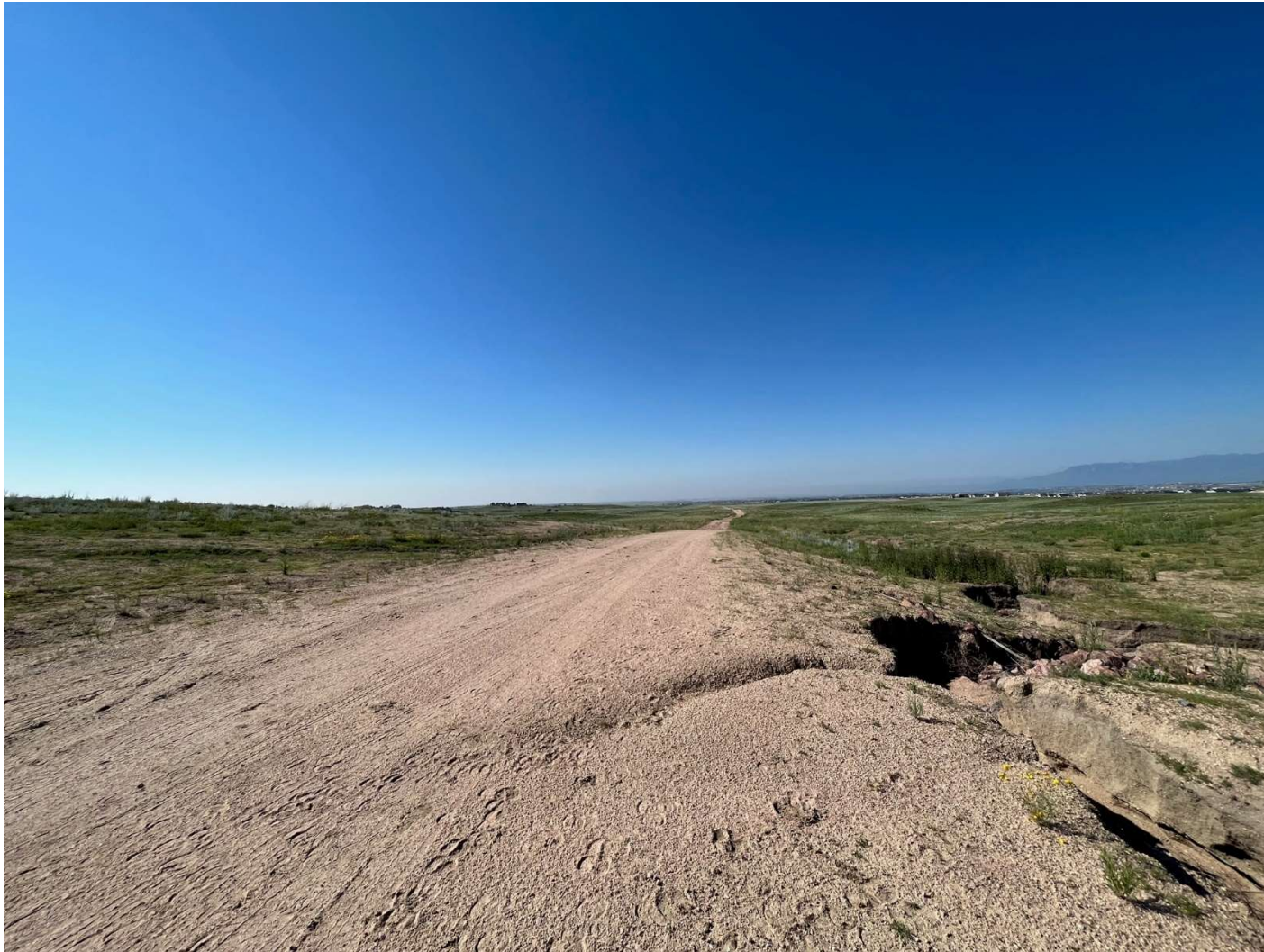
PHOTO 3 – Photo facing south of the construction road that runs through the center of the site. Upland areas are visible around this road, and an erosional feature can be seen on the right side of the photo.
