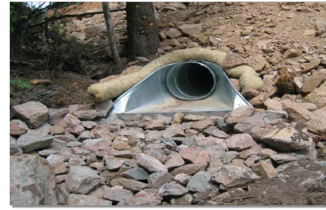
Photograph TOP-1. Riprap outlet protection.
