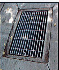
CDDOT Type C Grate (Close Mesh)
