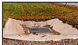
CUX01 Type C Inlet in Depression
