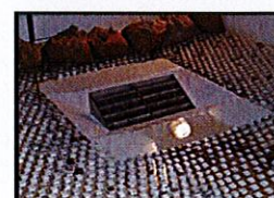
CDDOT Type D Inlet Parallel (30" Incline & Depressed)
