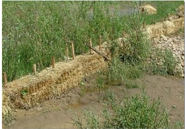
Photograph SBB-1. Straw bale barrier used for perimeter control. Photo courtesy of Tom Gore.
