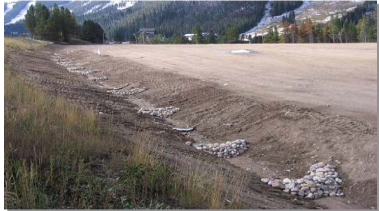
Photograph CD-1. Rock check dams in a roadside ditch. Photo courtesy of WWE.
