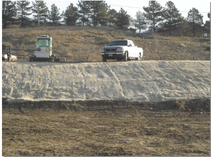
Photograph RECP-1. Erosion control blanket protecting the slope from erosion and providing favorable conditions for revegetation.
