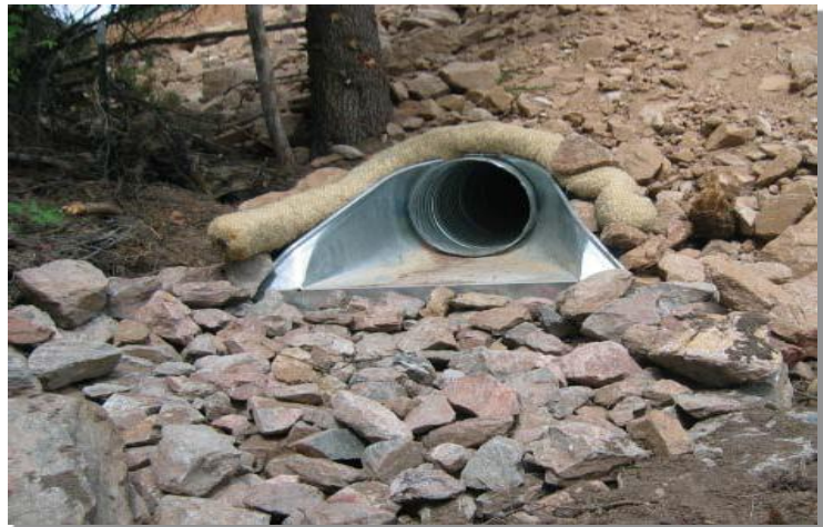
Photograph TOP-1. Riprap outlet protection.
