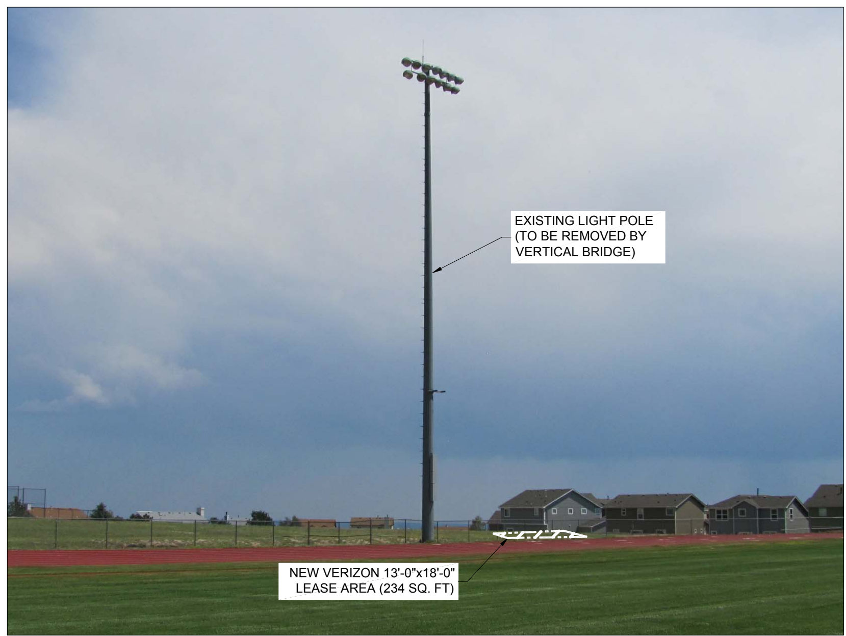
VIEW OF EXISTING STADIUM LIGHT POLE (LOOKING SOUTHEAST)
