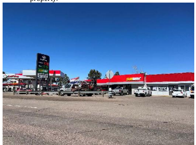
12. View of south adjoining filling station.
