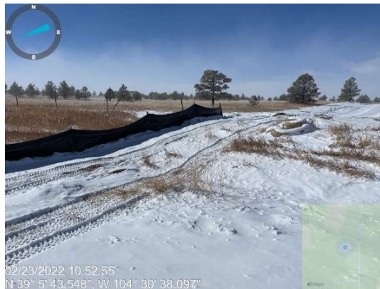
Silt fence control measure installed along site perimeter.
