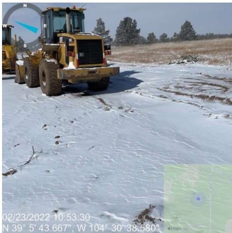
Construction equipment will be contained onsite for project.
