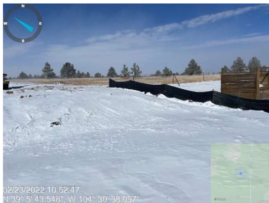
Silt fence control measure installed along site perimeter as per plans.
