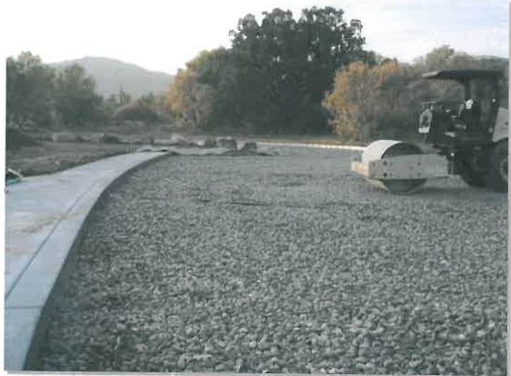
Photograph PPS-1. The reservoir layer of a permeable pavement provides storage volume for the WQCV. Photo courtesy of Muller Engineering and Jefferson County Open Space.
