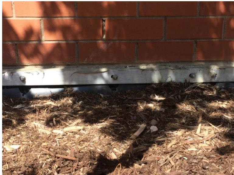
Photograph B-2. The impermeable membrane in this photo has ripped from the bolts due to placement of the media without enough slack in the membrane.
