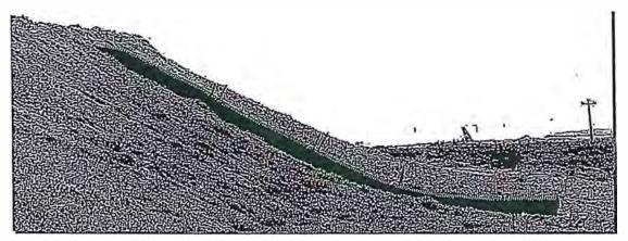
Photograph TSD-1. A temporary slope drain installed to convey runoff down a slope during construction. Photo courtesy of the City of Aurora.
