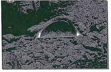
Photograph TOP-1. Riprap outlet protection.
