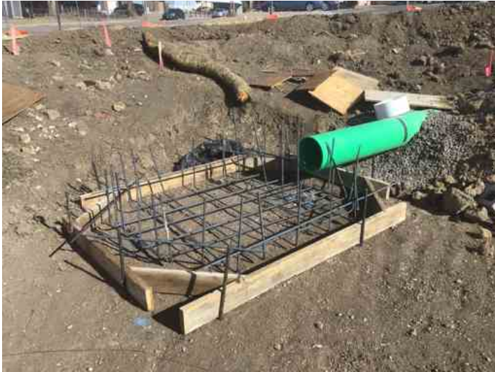
Reinforcement in place
