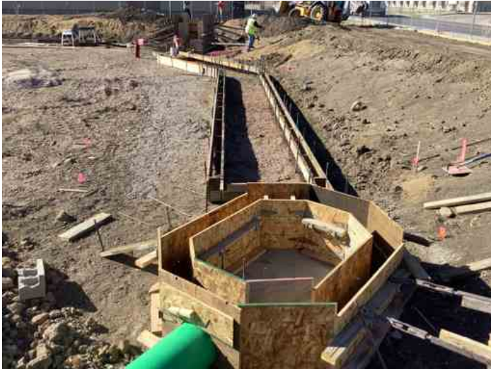
Forebay and storm detention channel
