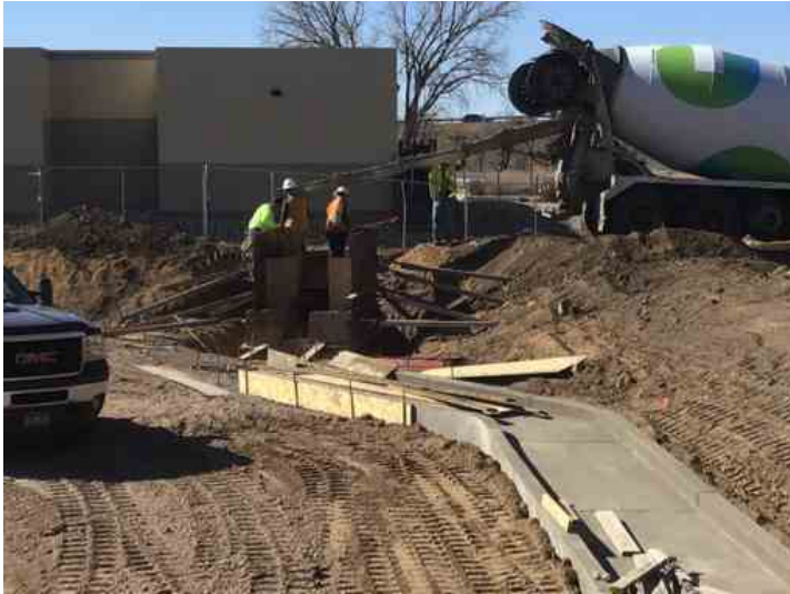
Concrete being tailgated in form
