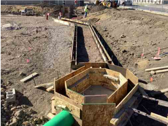
Forebay and storm detention channel
