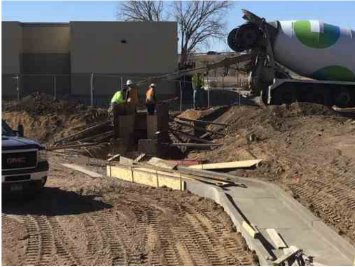
Concrete being tailgated in form
