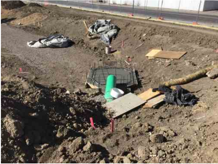
Concrete poured into form
