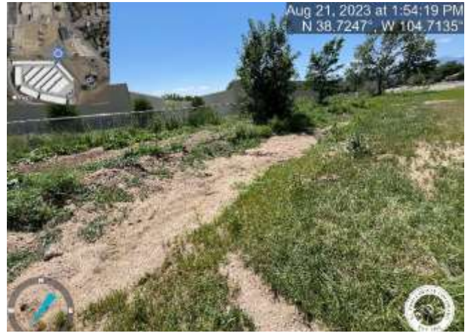
Photo 10: Remove sediment buildup within the grass-lined swale and reestablish vegetation in swale.
