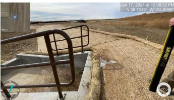
Photo 1: Tract F: Fine grade and seed with mulch the Runoff Reduction Area Open Space.
