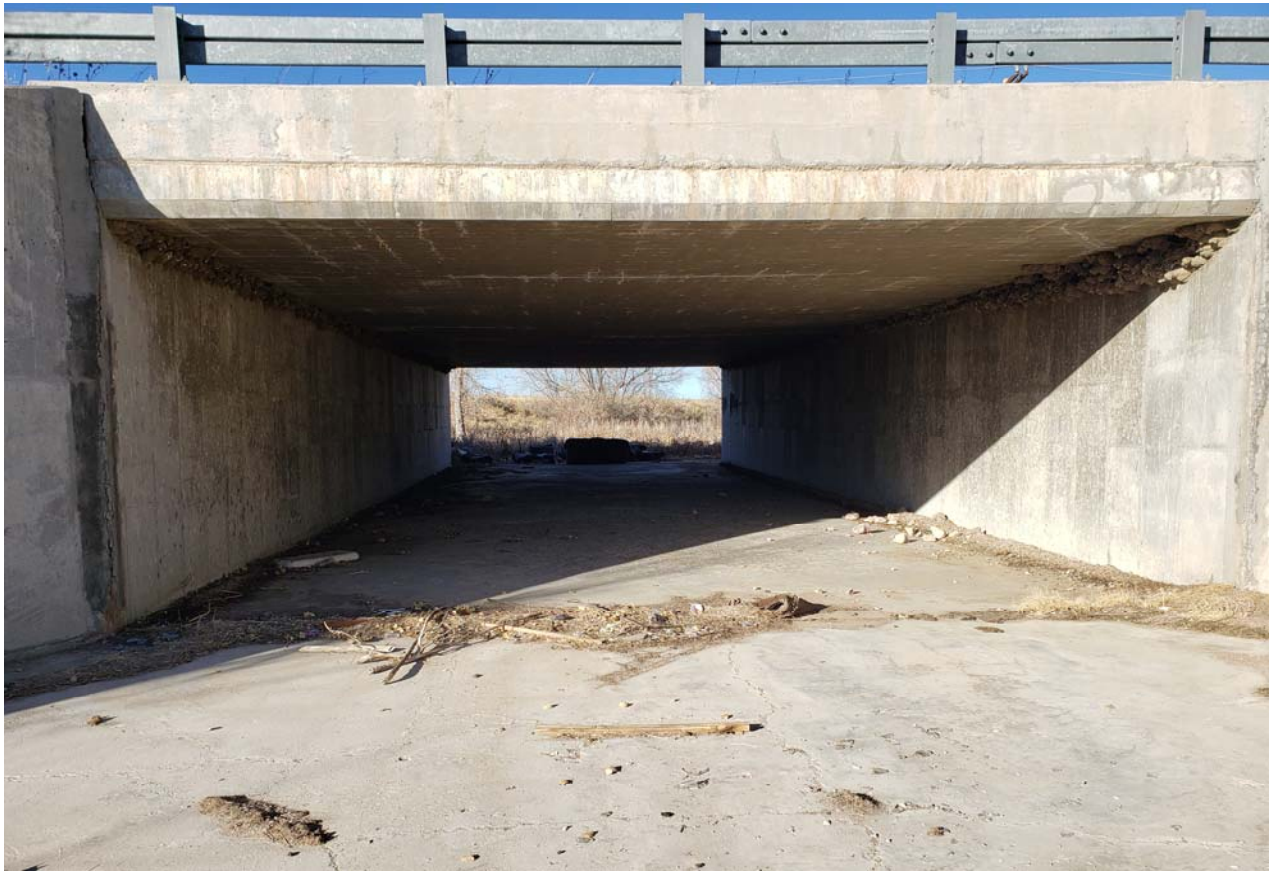
Figure 3-Existing 10' x 28' Concrete Box Culvert across Fontaine (Jimmy Camp Creek-West Fork)
