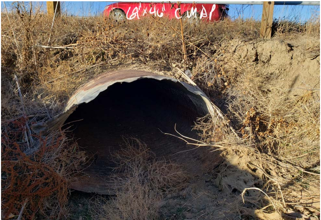
Figure 4-Existing 69" x 46" CMAP FMIC Culvert across Fontaine
