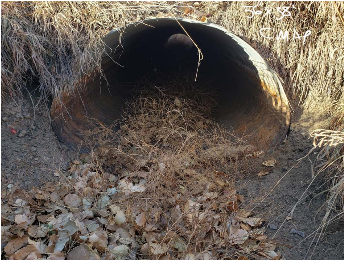
Figure 2-Existing 56" x 38" CMAP FMIC Culvert across Fontaine
