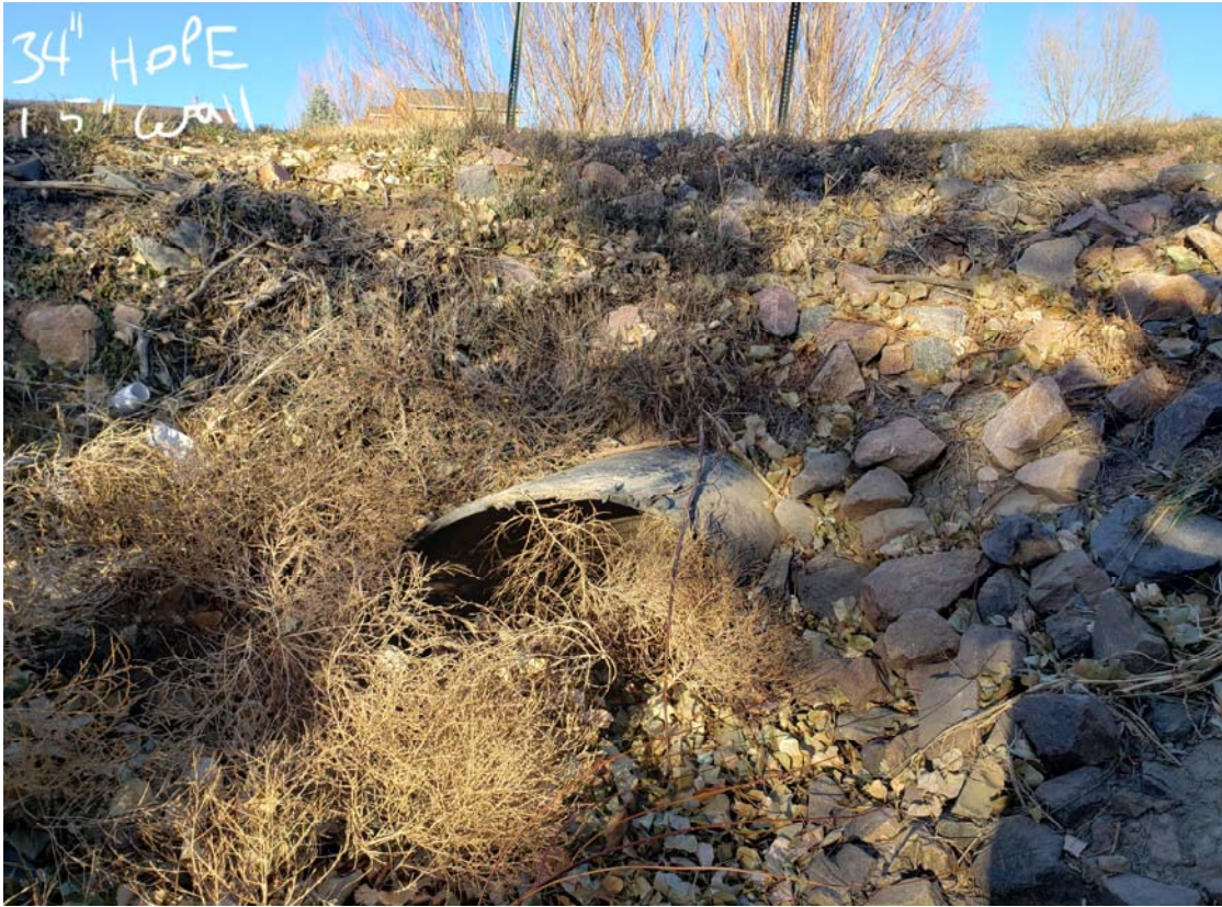
Figure 1-Existing 34" HDPE FMIC Pipe at Weeping Willow and Fontaine (Northeast of Corvallis)
