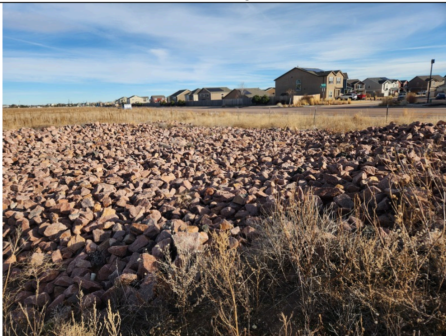
Rocks for storm water drainage on south side of site
