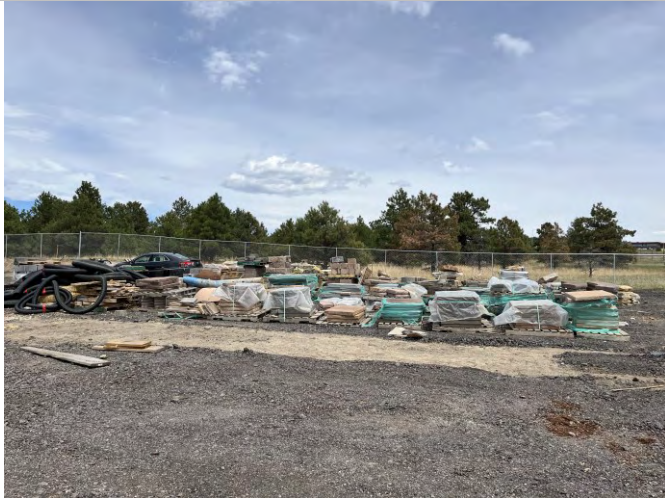
7. Material Storage to East of Building
