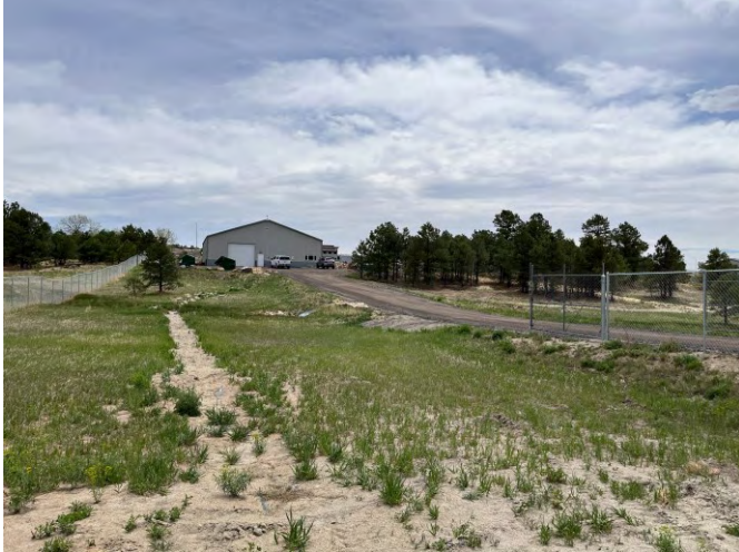
1. Building (Front) & Northwest Portion of Property
