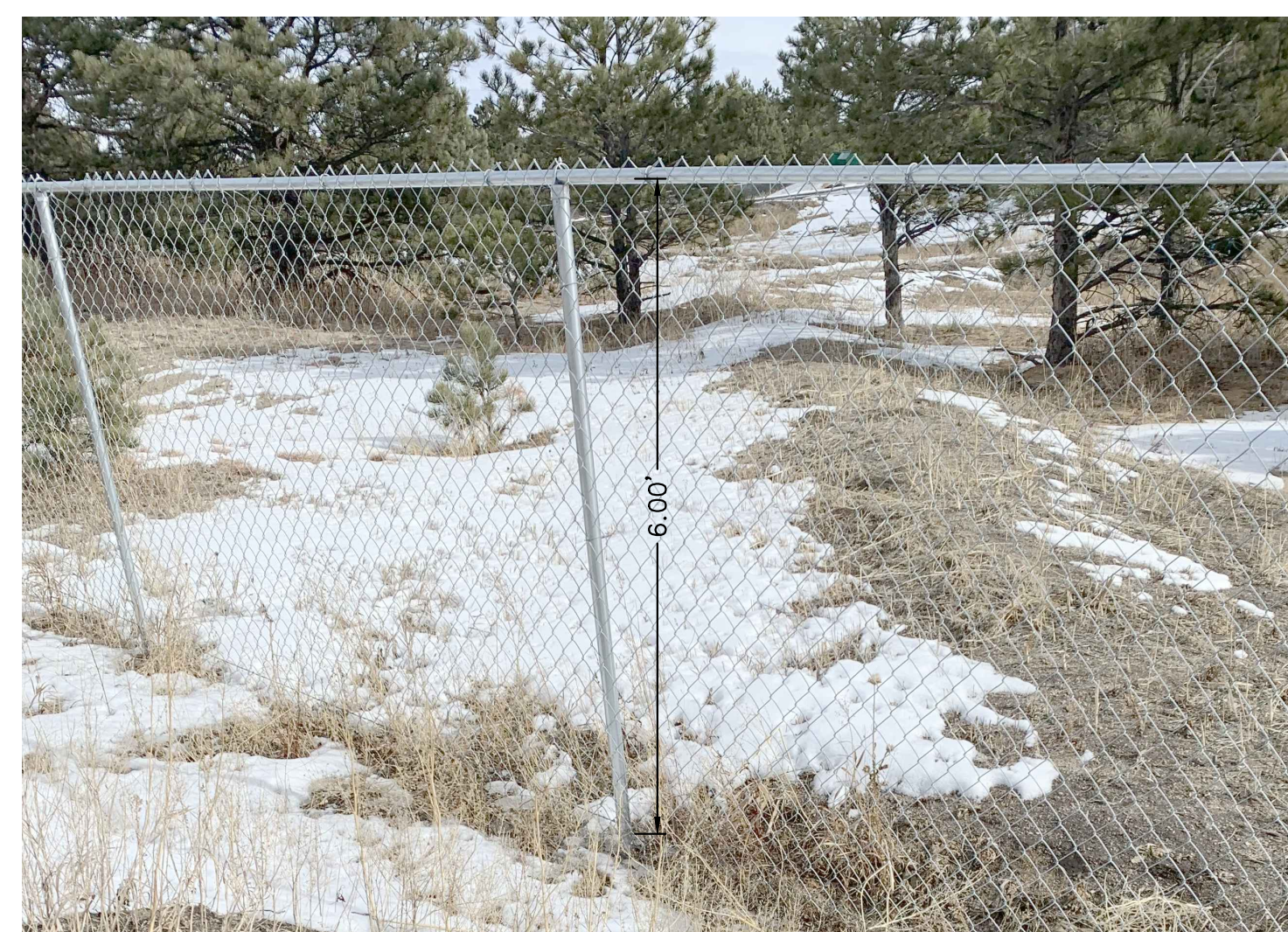
EXISTING CHAINLINK FENCE DETAIL
