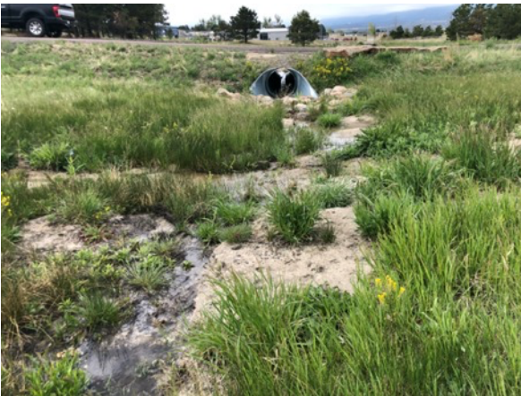
Photo #5 Wetland, north portion, view to north with driveway culvert outlet
