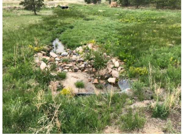
Photo #2 Site, culverts, view to south from driveway
