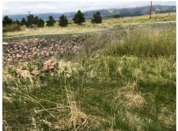
Photo #6 Wetland outlet riprap structure, south boundary of site
