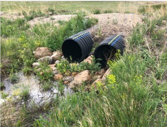
Photo #3 South culvert
