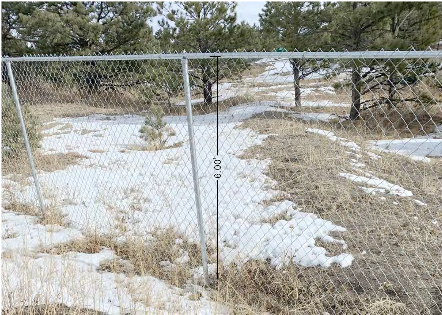
EXISTING CHAINLINK FENCE DETAIL
