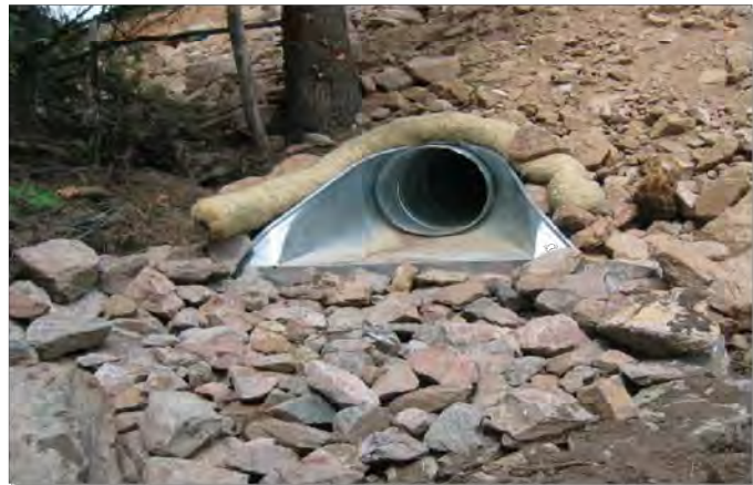
Photograph TOP-1. Riprap outlet protection.
