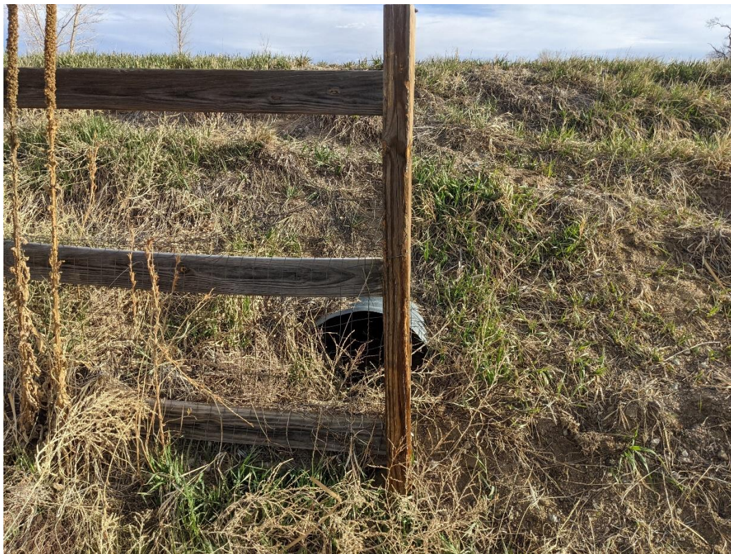
Figure 1: Storm Drain Culver Beneath Falcon Highway
