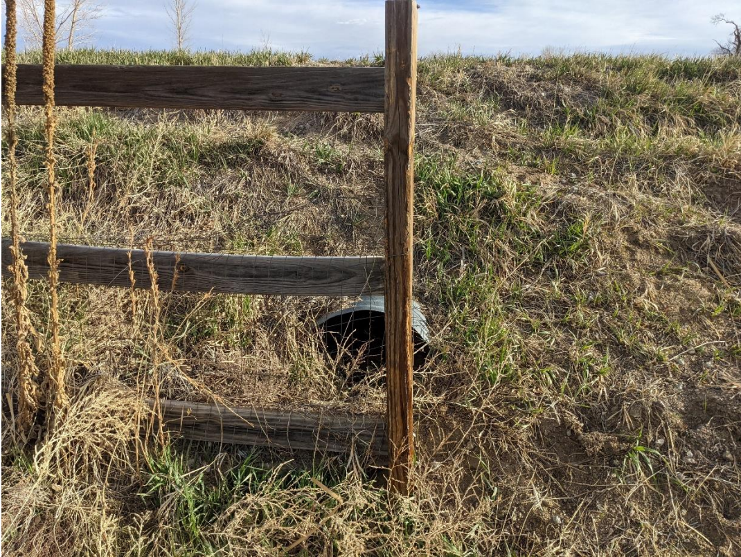
Figure 1: Storm Drain Culver Beneath Falcon Highway
