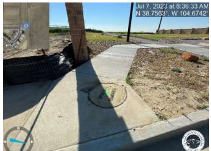
Photo 4: Example of marked stormwater inlet structure that needs to be cleaned of sediment and debris. Not all marked inlets are depicted in these photos.
