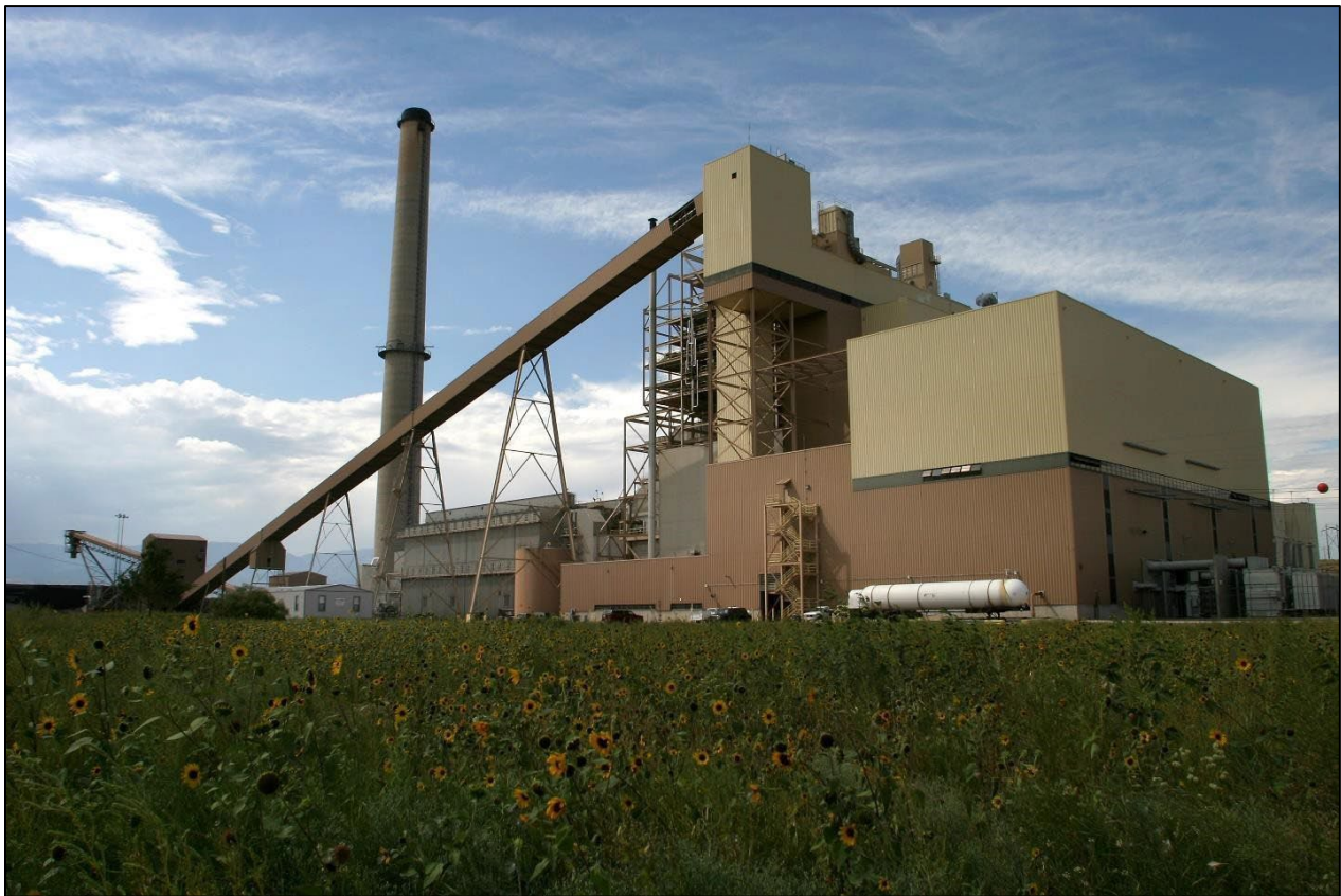
Figure A- 1: Ray Nixon Power Plant
