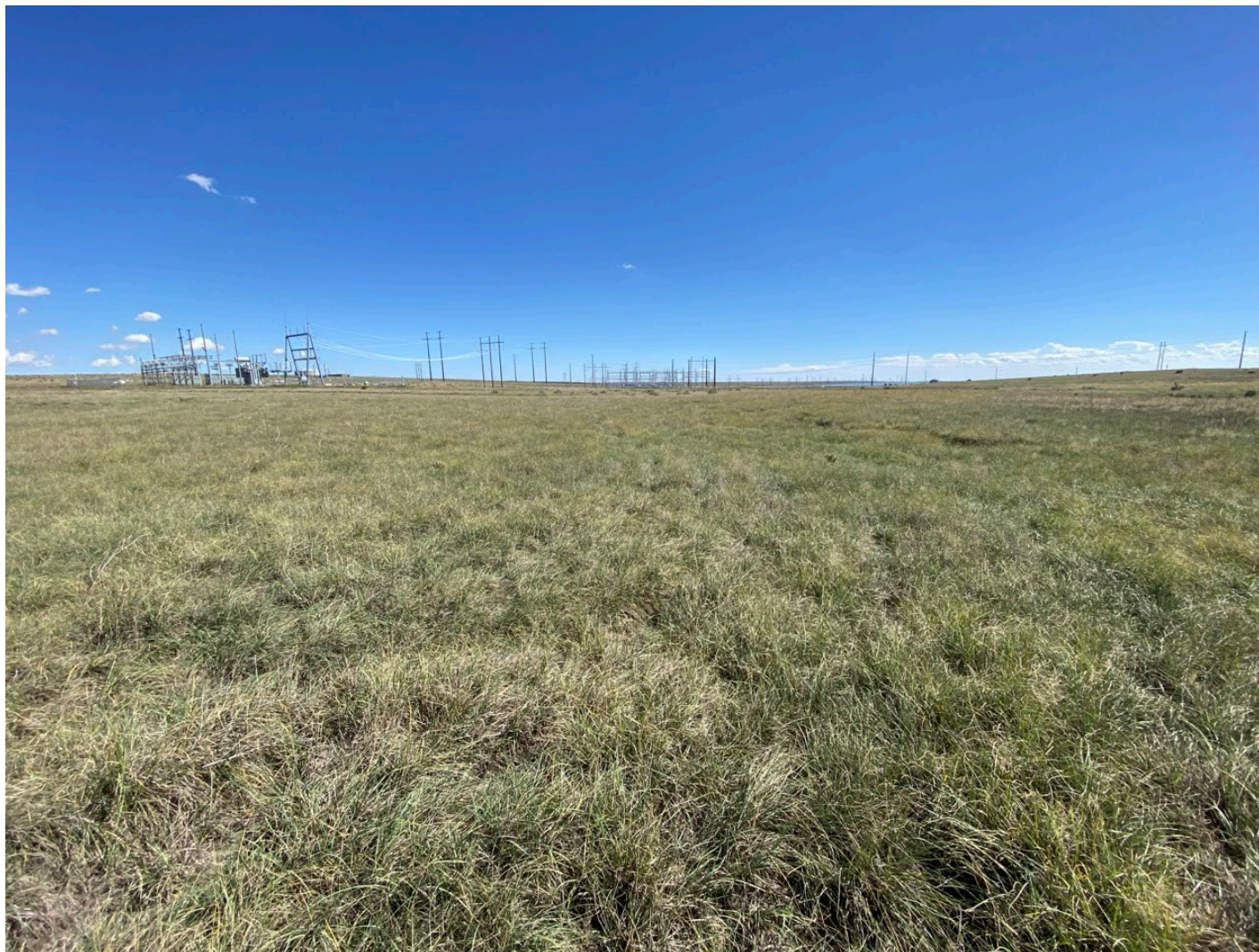
PHOTO 4 – Overview facing southeast of the typical vegetation found throughout the site, dominated by sand dropseed and blue grama. Existing infrastructure onsite can be seen in the background of the photo, including power lines and substation.
