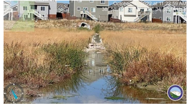
Photo 8: South trickle channel needs repair at Pond E
