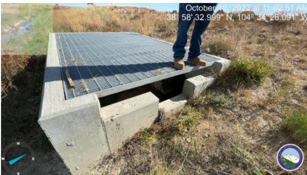
Photo 5: Weir notch was not built per plan at Pond E
