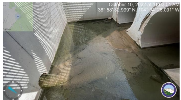
Photo 6: Cleanout of sediment at North outfall structure at Pond E
