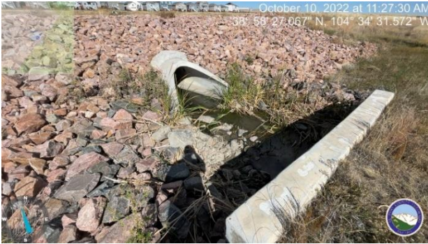
Photo 7: Riprap outlet protection inadequate at Pond E
