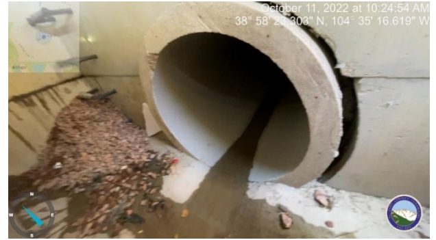
Photo 20: Inlets throughout filing need to be cleaned out and debris removed
