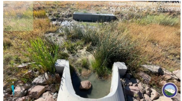
Photo 2: Riprap outlet protection is inadequate at Pond H outlet
