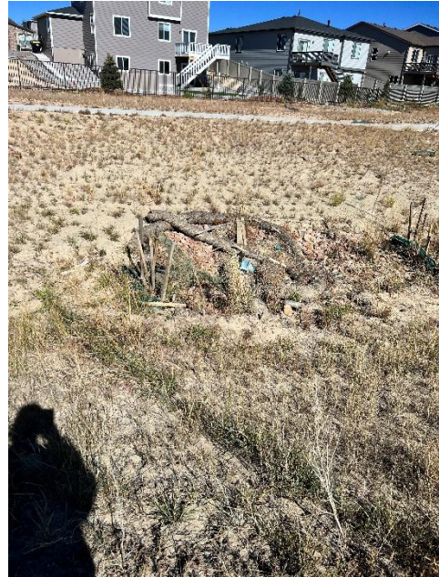
Photo 16: Storm #4 outlet needs to be cleaned and temporary BMPs removed.
