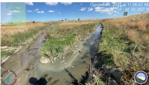
Photo 13: Trickle channel needs cleaned out at Pond E
