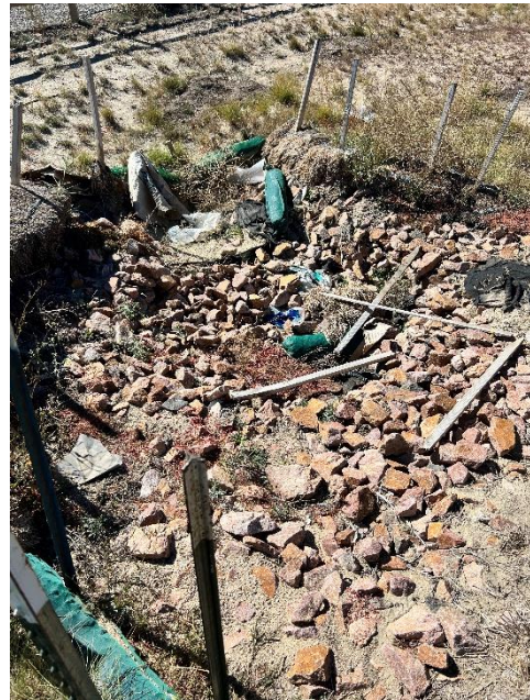
Photo 18: Storm #7 outlet needs to be cleaned and temporary BMPs removed.
