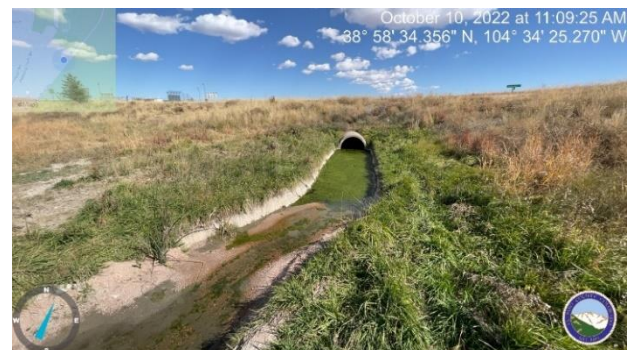
Photo 12: Excess standing water throughout Pond E. Northern most inlet pipe
