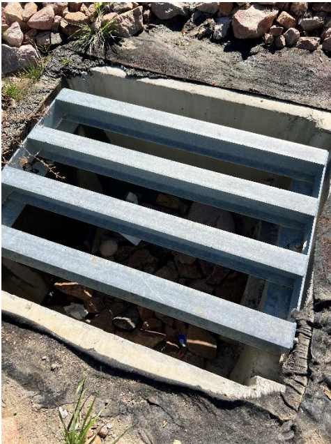
Photo 17: Storm #7 inlet needs to be cleaned out.
