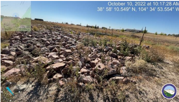
Photo 1: Remove weeds from spillway at Pond H
