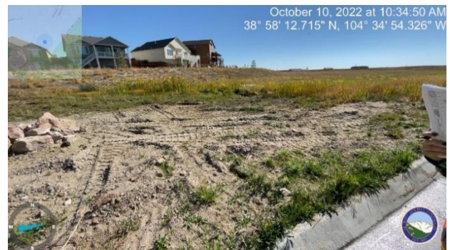
Photo 4: Mowing needed throughout Pond H. Seeding and stabilization needed.
