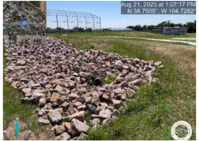
Photo 18: SE corner of building: Show riprap pad on As-builts.
