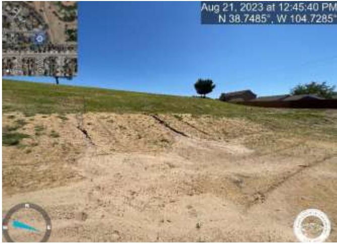
Photo 7: Pond: Grade out riling along pond slopes and stabilize in various areas.
