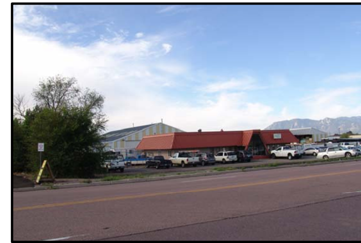
SITE PHOTO - VIEWING SOUTH
