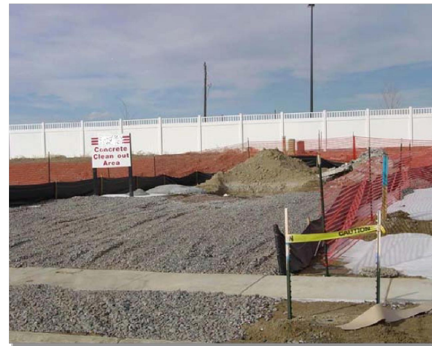
Photograph CWA-1. Example of concrete washout area. Note gravel tracking pad for access and sign.
