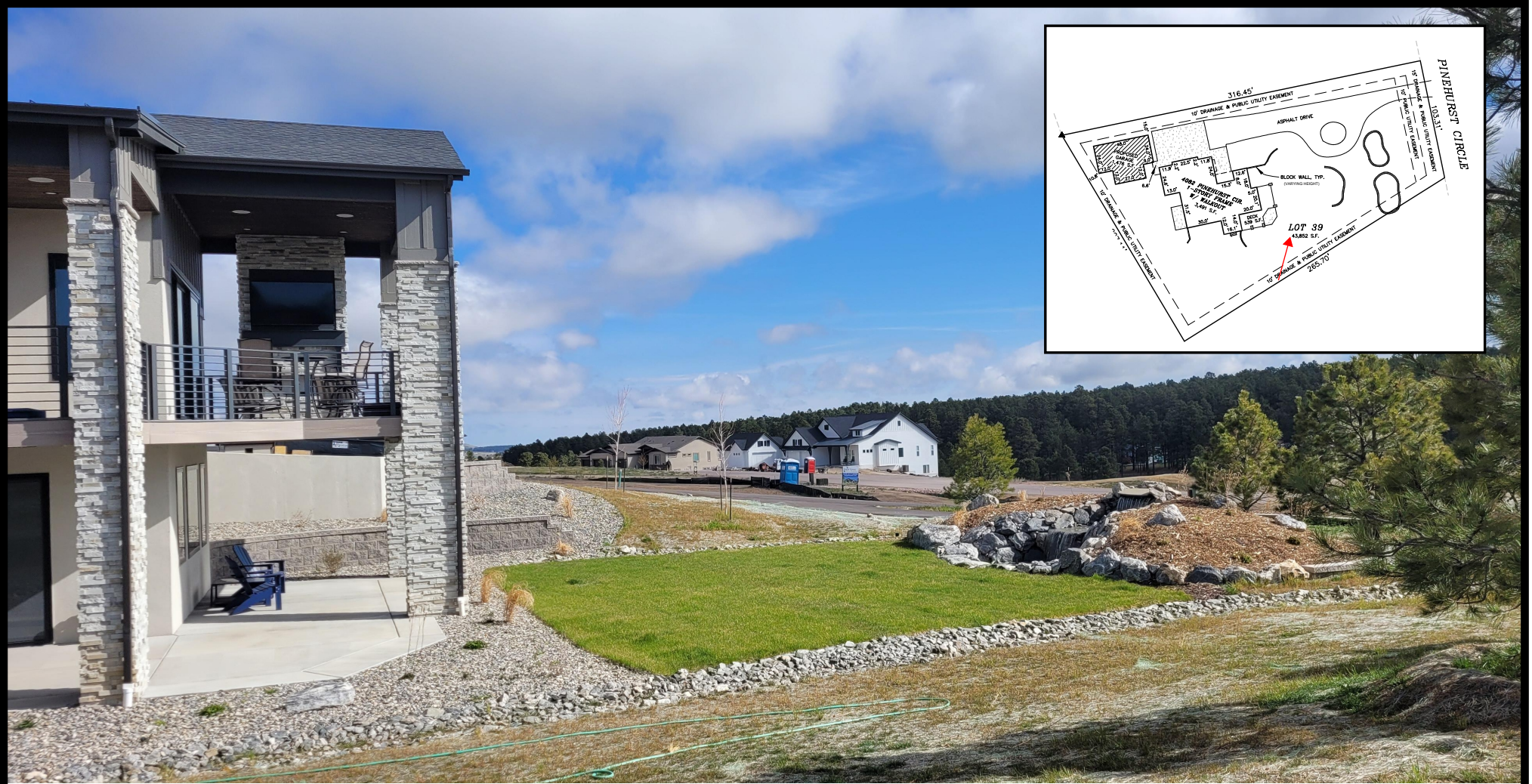
Landscape area that would need to be removed if setbacks were met (Note drainage area that would need to be rerouted, closer to trail)
