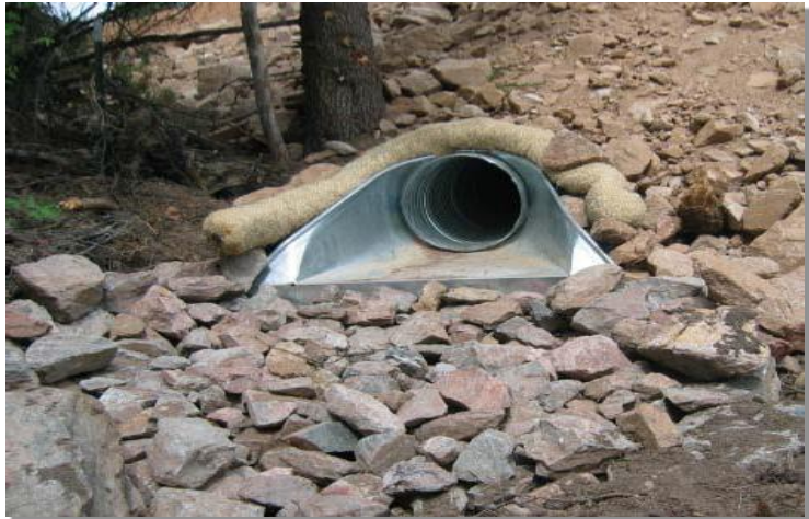
Photograph TOP-1. Riprap outlet protection.
