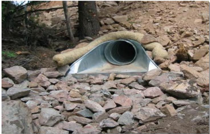
**Photograph TOP-1.** Riprap outlet protection.
