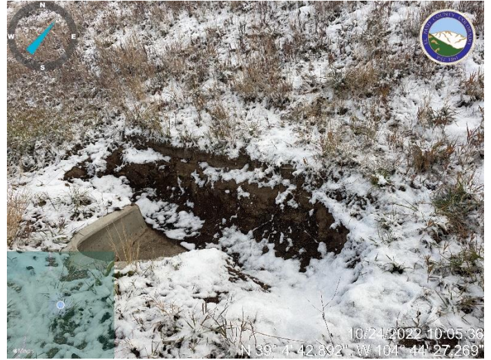
Photo 2: Field fit culvert with riprap on upgradient side where straw bale barriers were removed to ensure positive drainage in ditch along Settlers Ranch Rd.
