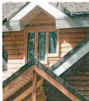
Enclose eaves and soffits.
