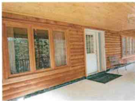
Use a concrete patio instead of a wooden deck and rubber mats instead of natural fiber.
