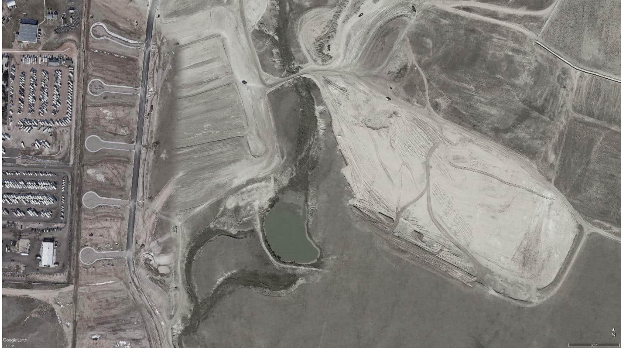
Figure 5 – Road Detention and Pond #3
