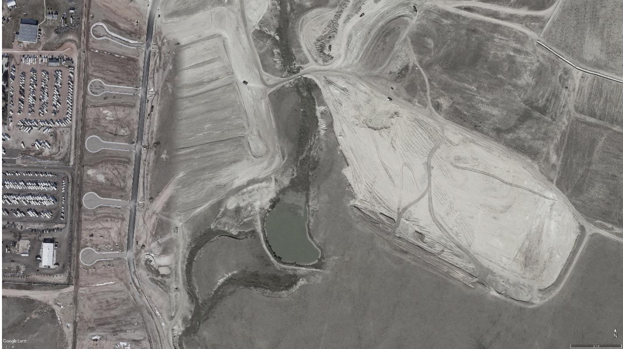
Figure 5 – Road Detention and Pond #3
