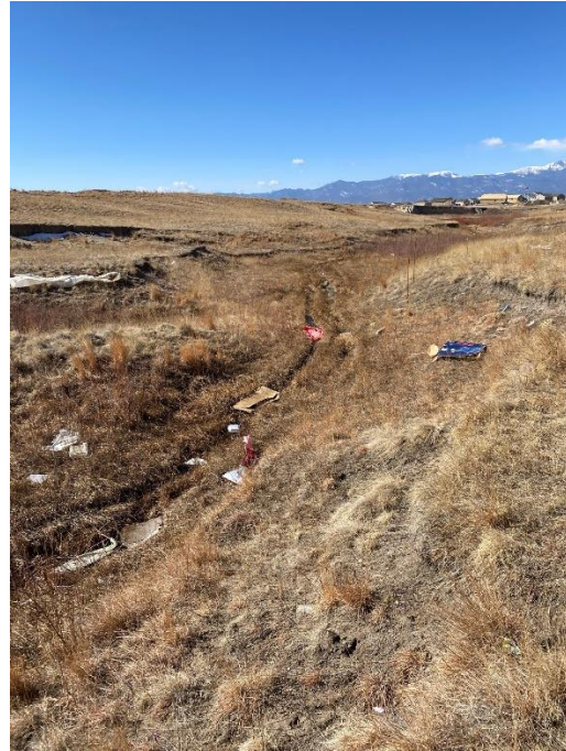
Figure 9 – Confined Valley, Limited Bank Erosion
