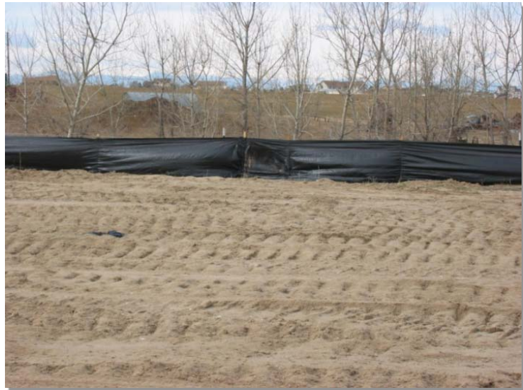
Photograph SF-1. Silt fence creates a sediment barrier, forcing sheet flow runoff to evaporate or infiltrate.
