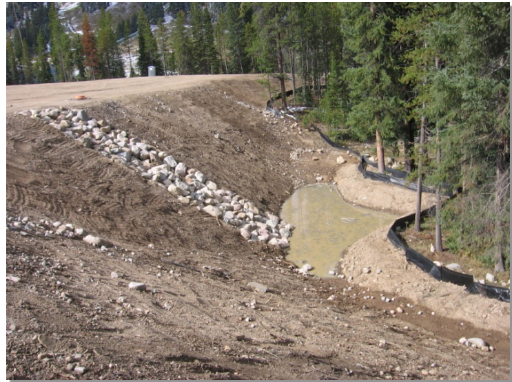
Photograph SB-1. Sediment basin at the toe of a slope. Photo courtesy of WWE.
