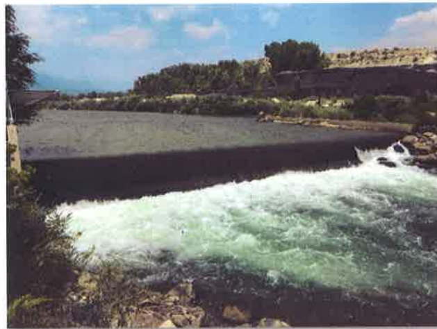
Arkansas River Diversion Structure near Salida, CO
