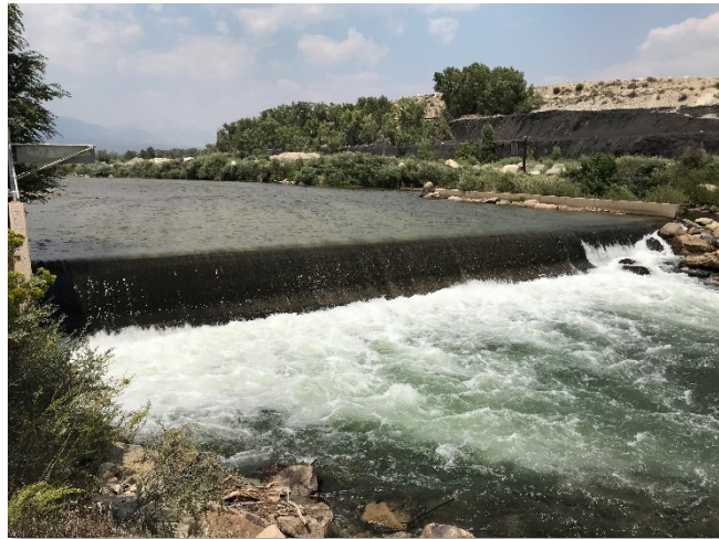
Arkansas River Diversion Structure near Salida, CO
