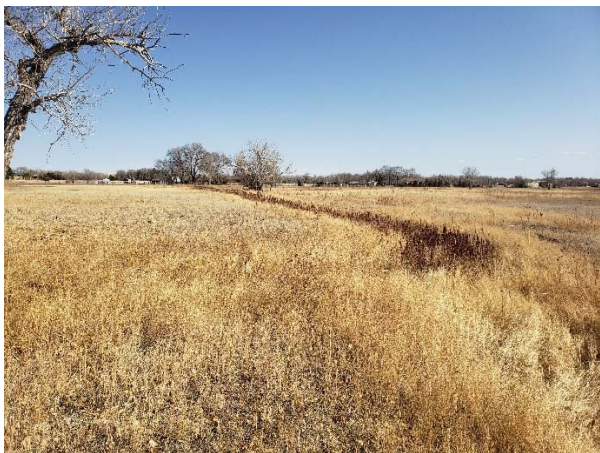
WF Jimmy Camp Creek invert facing north.
