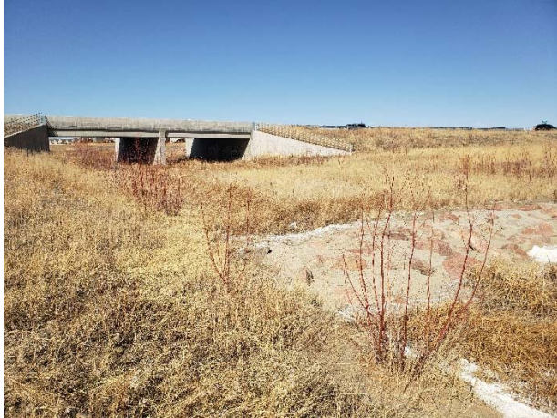
WF JCC Mesa Ridge Parkway Bridge facing North
