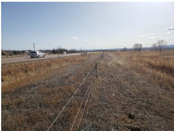
Invert along Marksheffel Rd. facing southwest.
