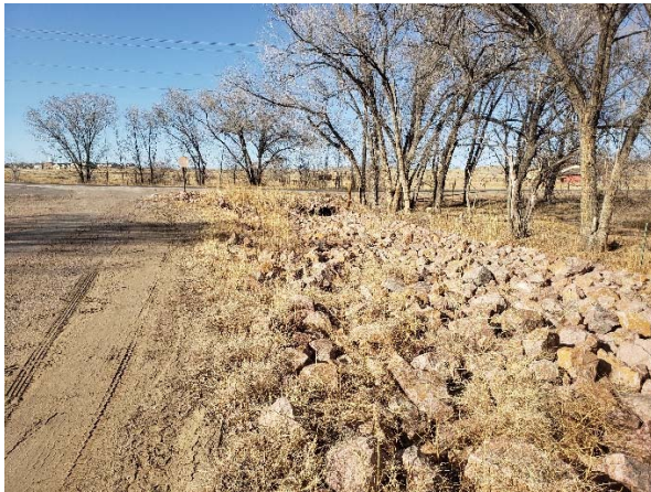
DP 1250 C&S road crossing and channel to north
