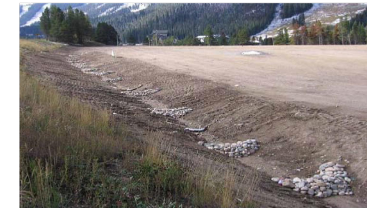
Photograph CD-1. Rock check dams in a roadside ditch. Photo courtesy of WVE.
