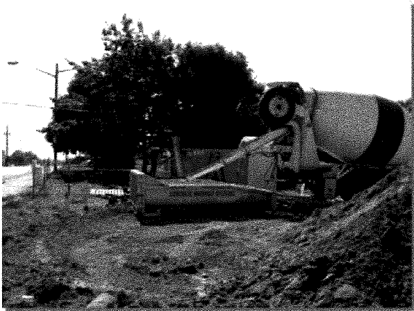
Photograph CWA-2. Prefabricated concrete washout. Photo courtesy of CDOT.
